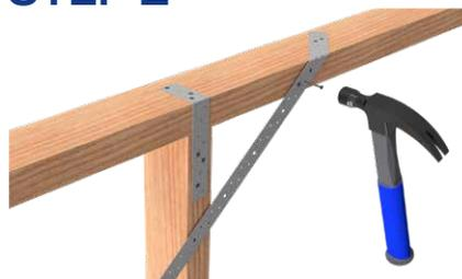
Wrap VUEBRACE over the top of the plate and nail brace to the top plate using 4x 30mm x 2.8mm Ø VUETRADE Galvanised Timber Connector Plate Nails (as per Fixing Detail B of the TDS - see note for Fixing Detail A)
