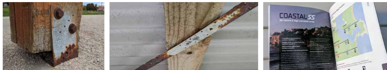
Above: Examples of corroded timber connectors installed in an area which is classed as Severe Marine.
